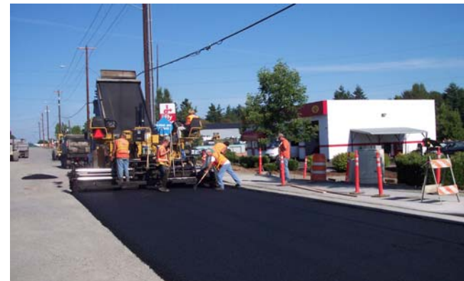
Total street section reconstruction Beavercreek Road
