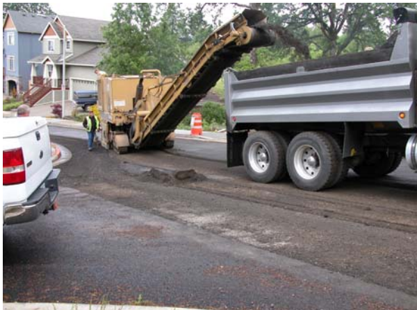
Cold plane pavement removal (milling)
