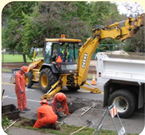
**Replacement of aging components in the drinking water distribution system is necessary to maintain good water quality and system reliability.**
