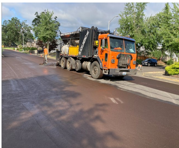
Slurry Seal Treatment
