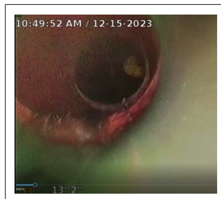
Tree root intrusion in pipe
