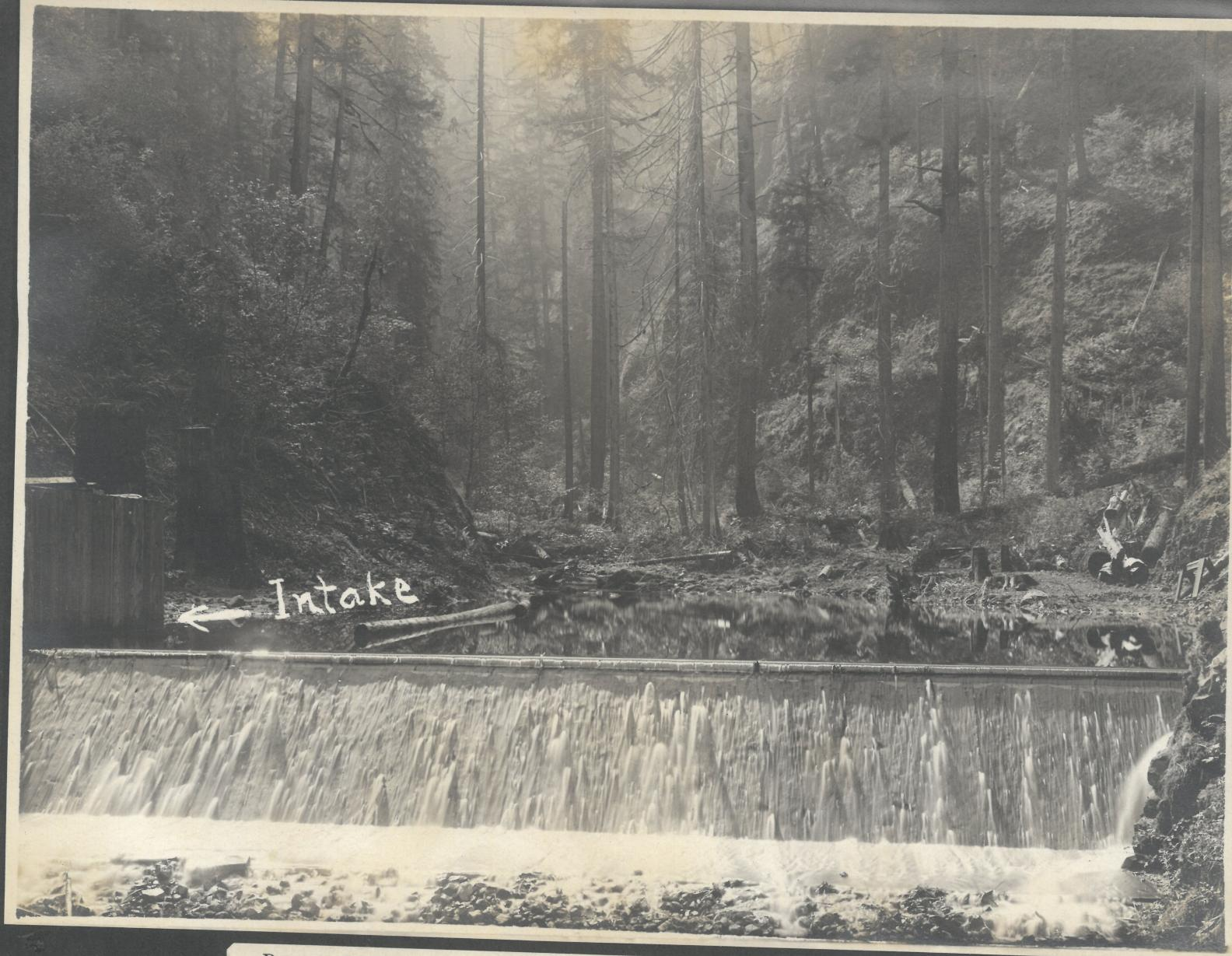
*Dam and Intake, where water enters a twenty-inch pipe through a wire screen.*
