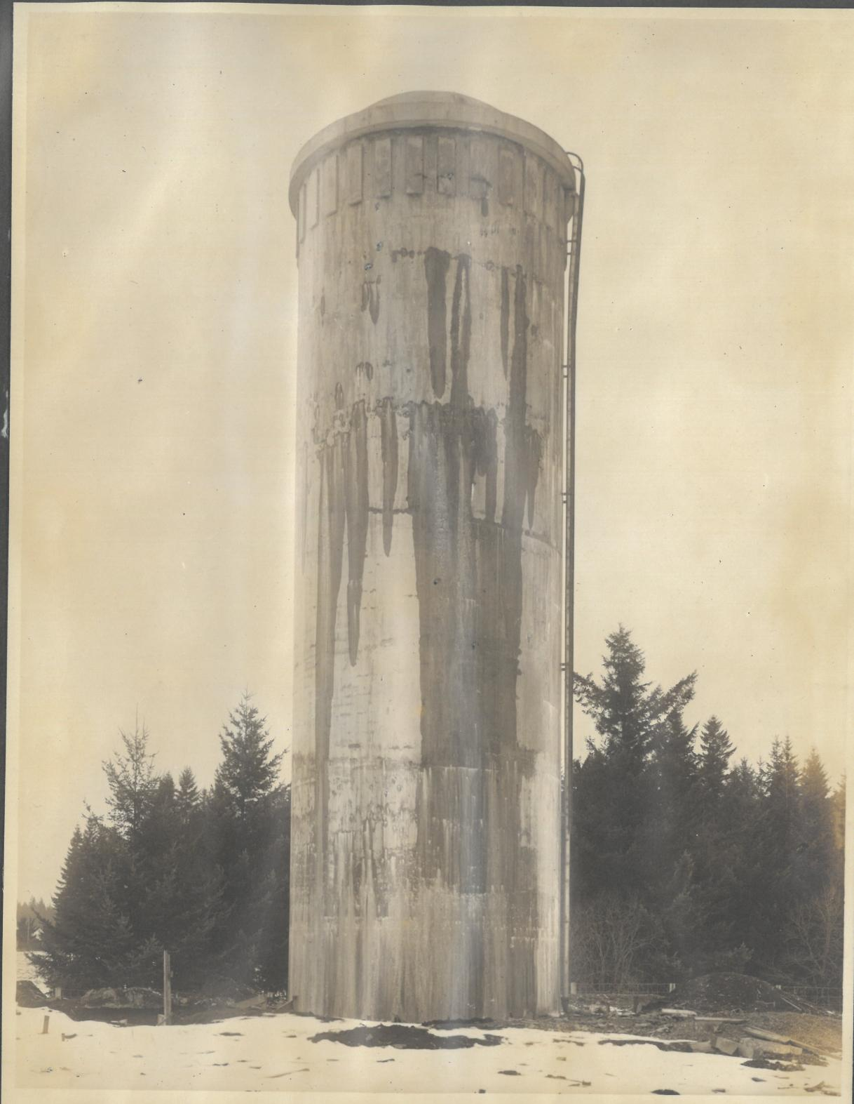
West Linn's stand pipe when completed, capacity 60,000 gallons.
