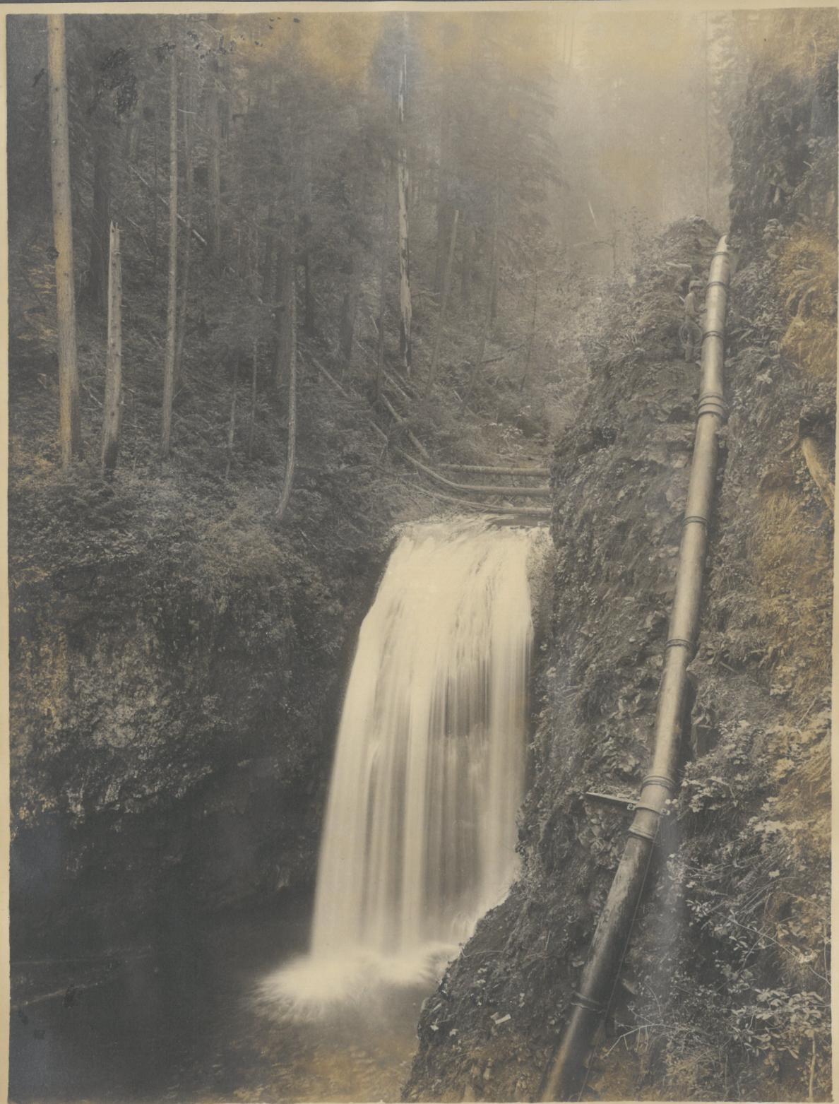
*Lower Fall, showing pipe line anchored to precipice.*
