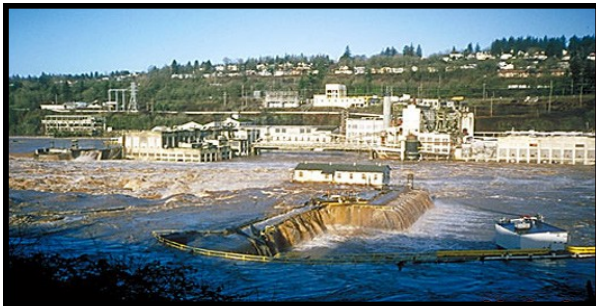
Willamette Falls 2/10/1996—photo courtesy of Lew Scholl
