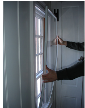
Interior storm panel.
