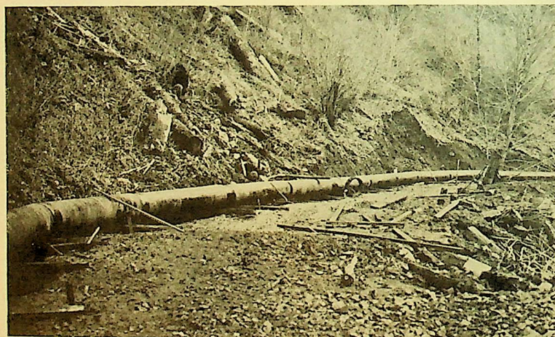
Twenty-four inch Steel Welded Pipe Ready to Place in Trench, from Intake to Settling Basin, 665 feet.
