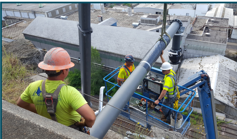
Installing new water main
