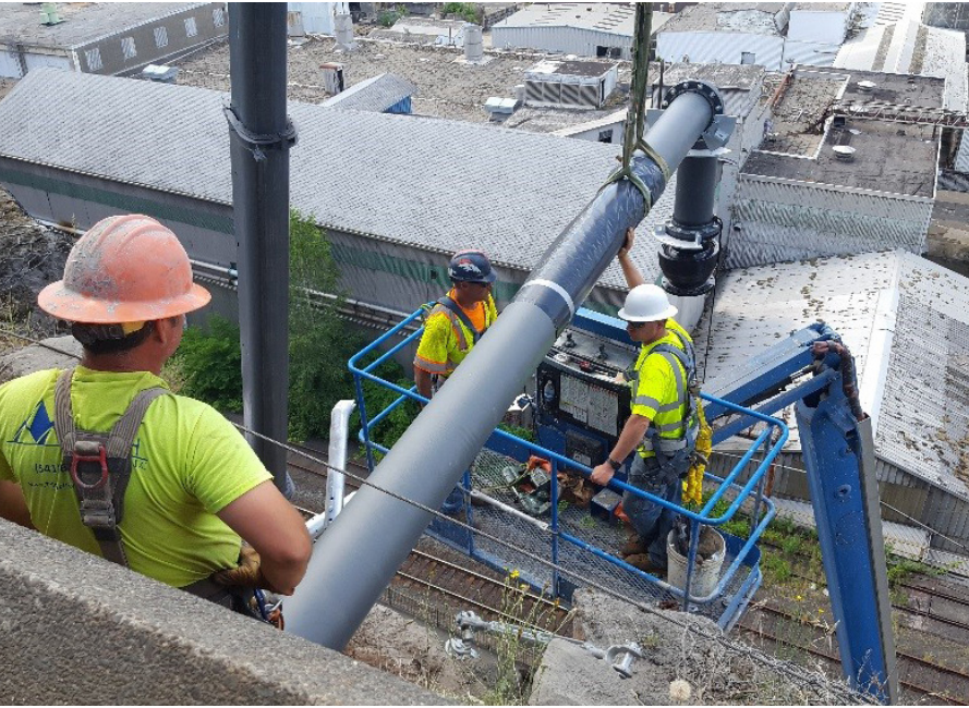
Installing upper pipe section and ball joint
