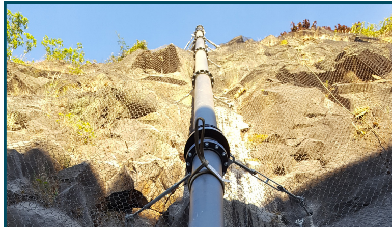
Base support for new water main
