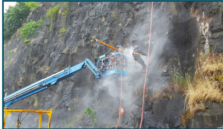
Drilling pipe support anchors
