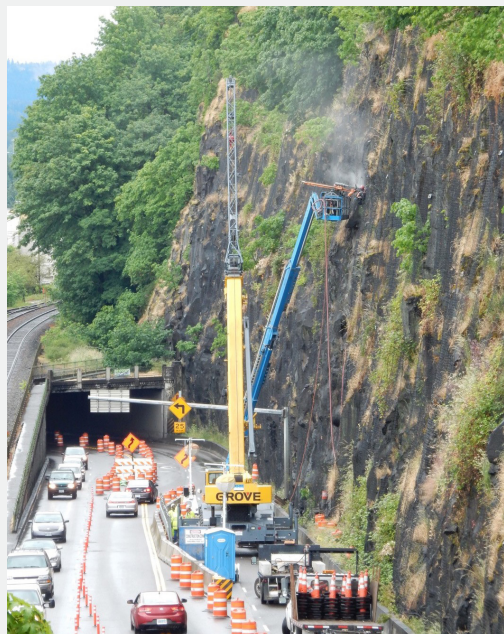
The proximity between the project area and the tunnel limited the allowable work zone.
