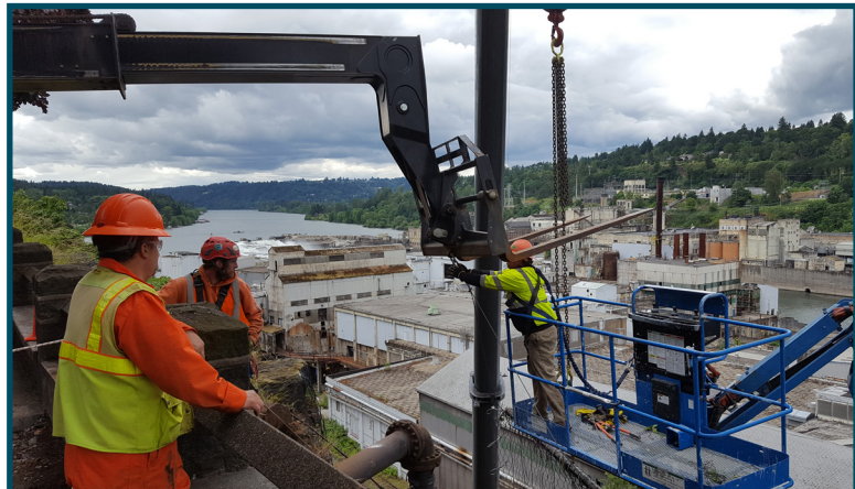
Preparing to remove existing water main
