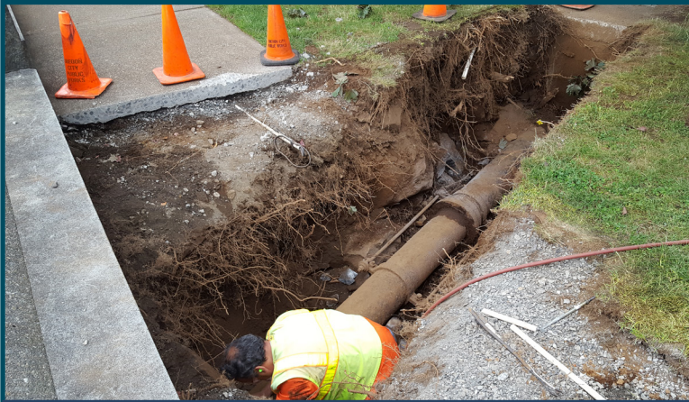
Excavation of existing main at top of Bluff
