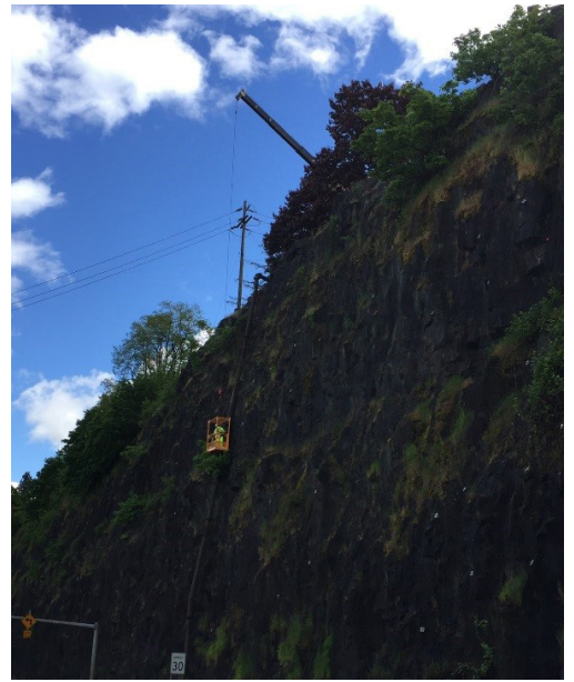
Pre-fabrication survey of existing pipe and rock face profiles
