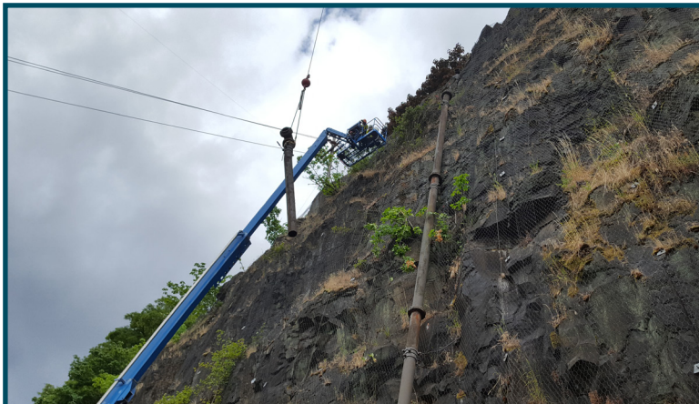
Removal of existing water main
