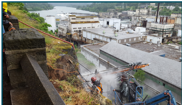
Drilling pipe anchors
