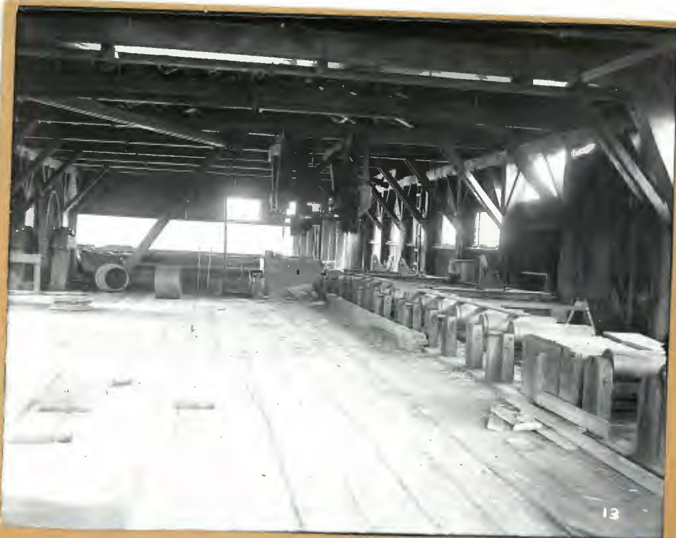
Interior Broughton Saw Mill looking to River 8/13
