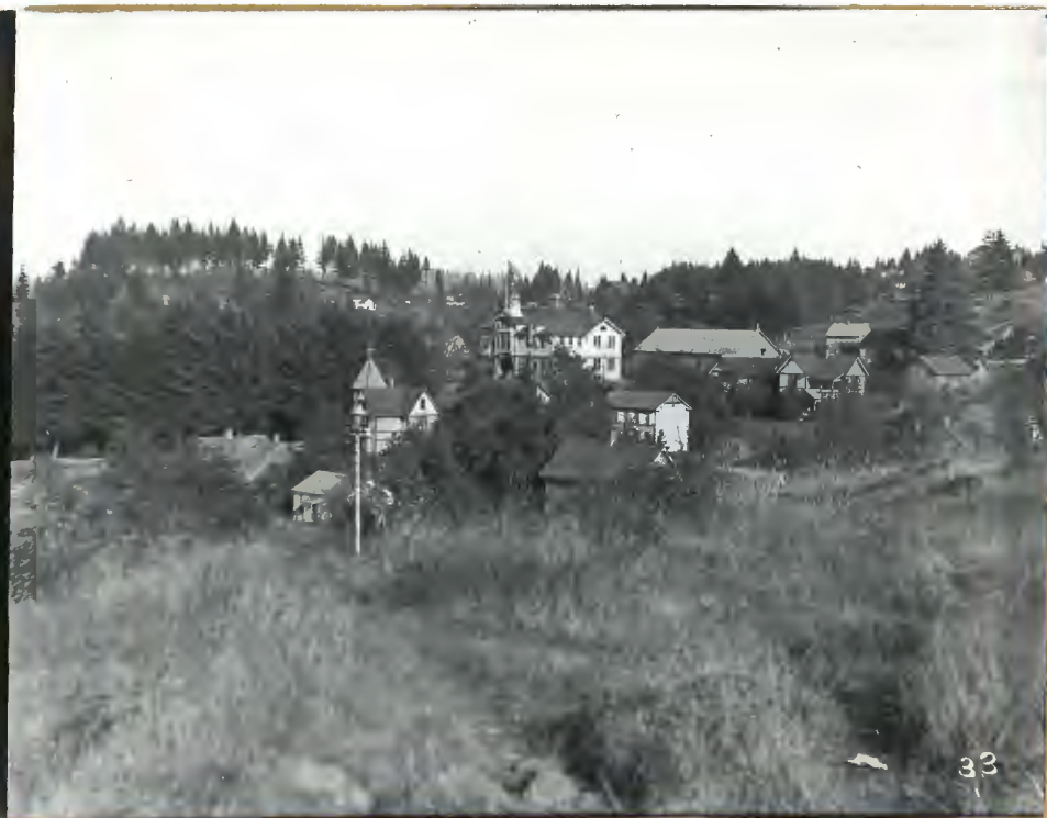
Barclay School & Gymnasium
