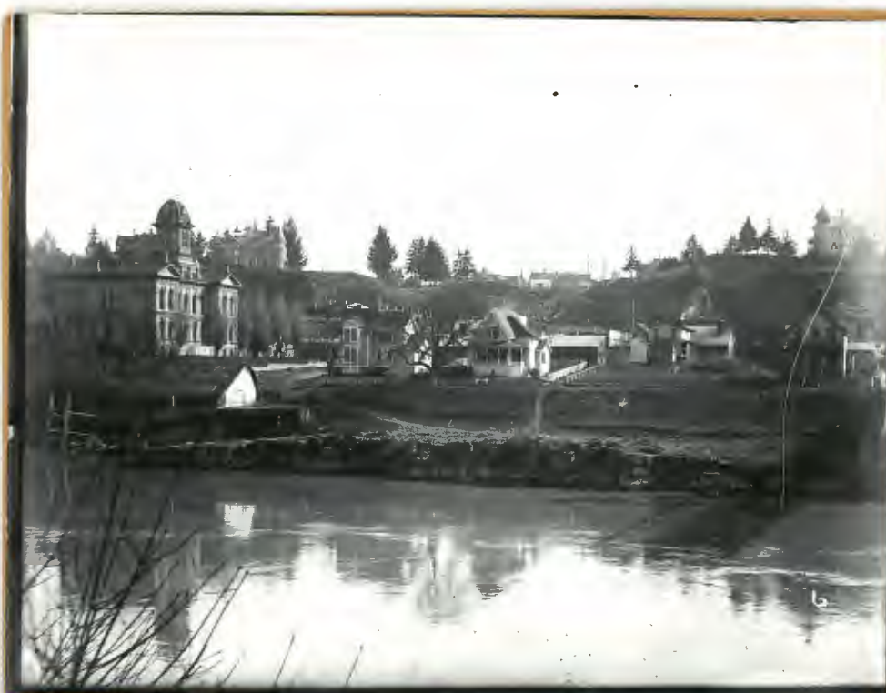
Rth St Dock at 8th + Water to 7th
