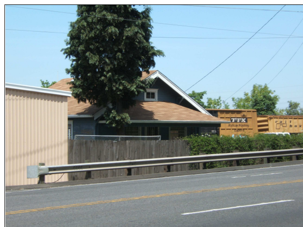
South facade, looking north
