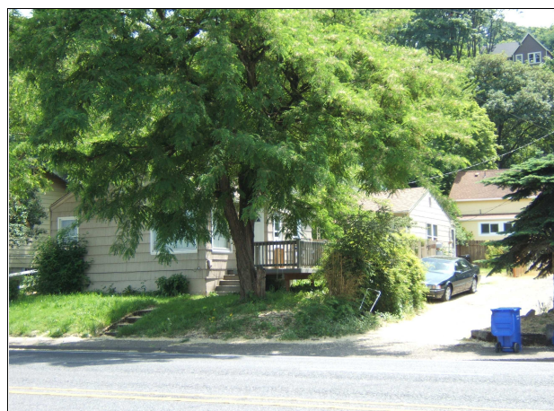
Northwest facade, looking southeast
