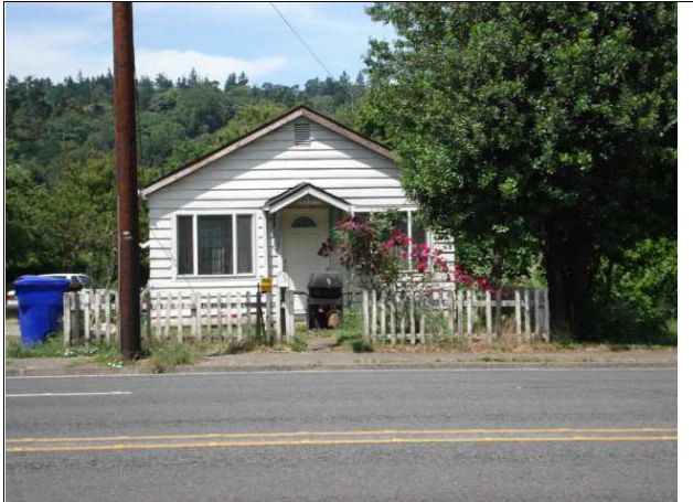
South facade, looking north
