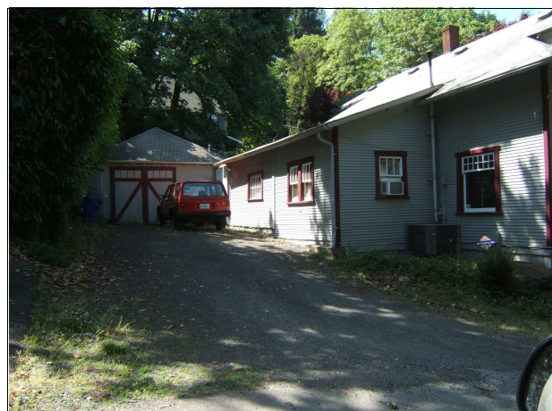
North facade, looking south
