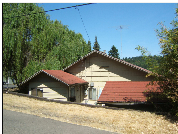
South facade, looking north
