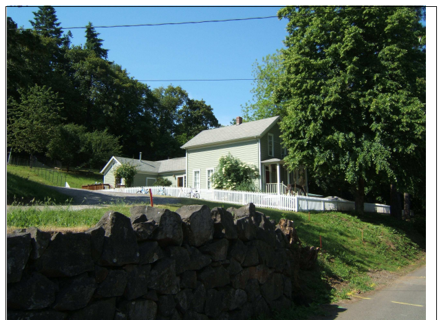
Northeast facade, looking northwest
