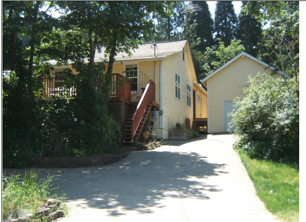
Northeast facade, looking southwest
